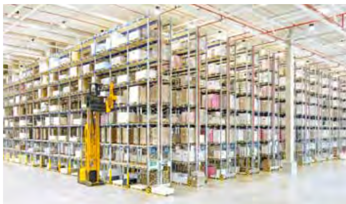
Highbay pallet racking
